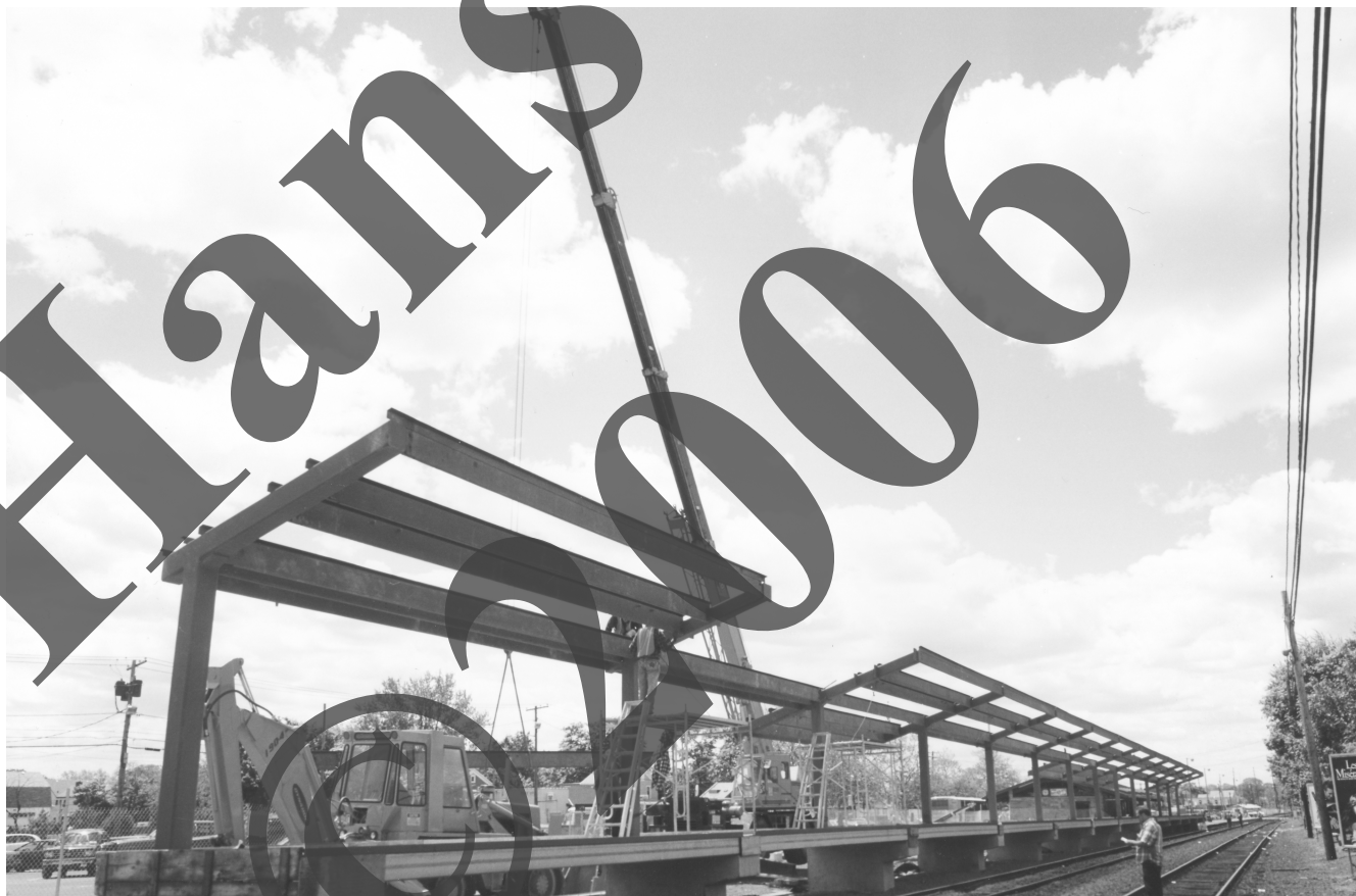
Railroad platform under construction. This new type platform was needed to accommodate the new diesel – electric trains coming into service.
