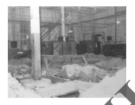
After all the machinery, foundations and other obstructions were removed, a new concrete floor was poured.
