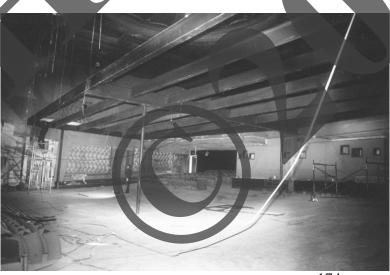
A view of the rear section of the theater. All these long i-beams that supported the extended balcony had to be removed.
