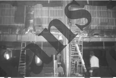
The conversion of the theater to a triplex did much damage to the interior. Here the dividing wall and the large I-beams supporting the balcony are being removed.
