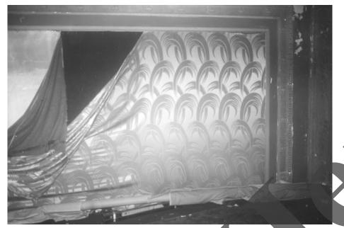
During renovations of the theater the walls were covered with new material without removing the old wall panels. These panels apparently are the original wall coverings, which appeared after other layers were removed.
