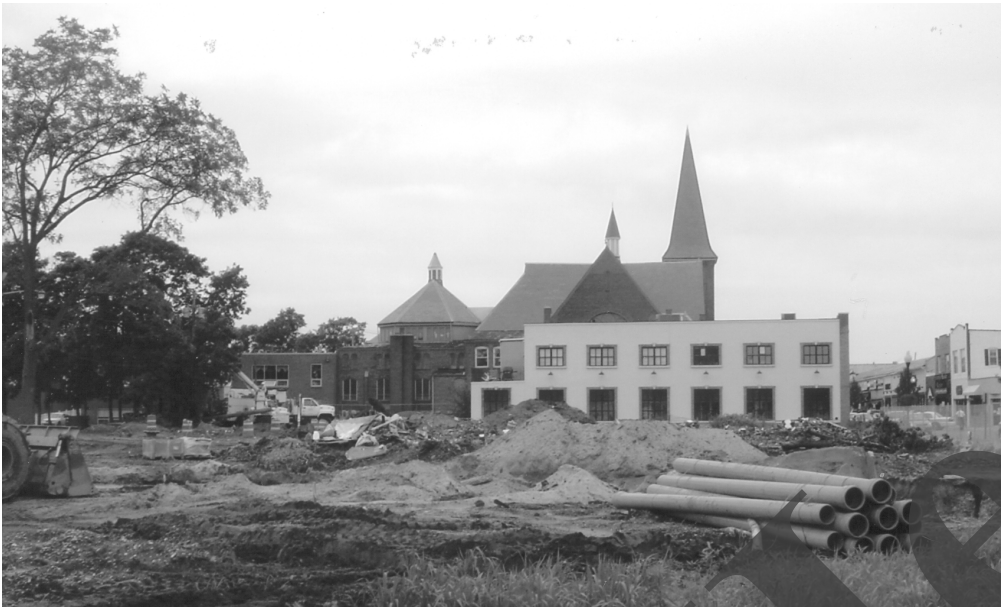
A view of the work in progress. The buildings on the right are on South Ocean Avenue and the Methodist Church is in the background.
