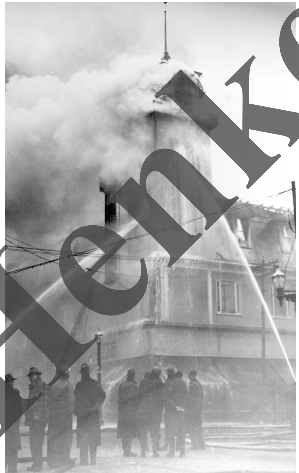
Firemen fighting the fire, January 9, 1946. The water cannot reach the fire inside the tower effectively.
