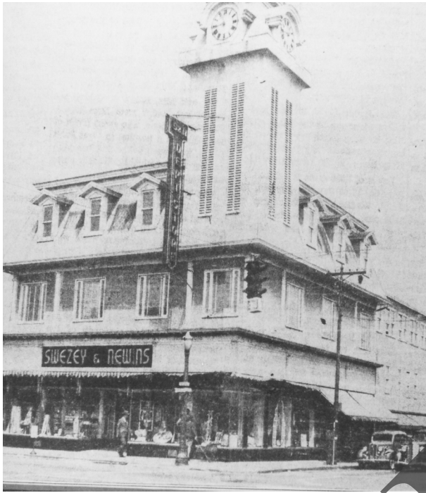
The Swezey and Newins Department Store in the 1930's. The tower had been changed from the original look by enclosing the sides and the windows with siding material, a fact that complicated the fighting of the fire in the tower in 1946.
