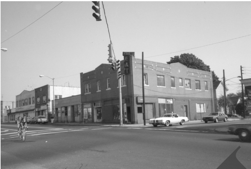
The southeast corner of Main Street and West Avenue in August 1981, site of the future Sixth District Court building.
