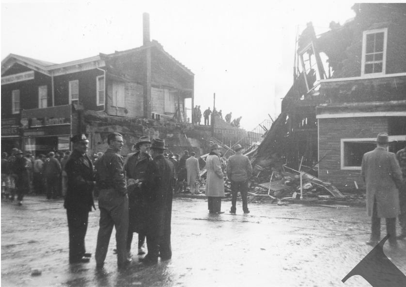
The Main Street section of the Mills Building after the fire. The building on the left survived the fire thanks to the great effort of the firemen and it is still standing today. This $1,000,000 fire destroyed the Woods Jewelry Store, the Glenda Lyn shop, the Miles Shoe Store, Cantors Dress Goods, Muriel Modes, Falkoff Shoe Store, Blum's and the Stuart Drug Store.
