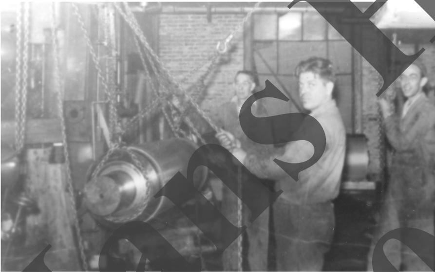
Some of the machinery in the mill was dismantled previous to the closing. Stan Edwards, E. Gregory, and A. LeBranch are removing a Perkins Roll for packing and shipping. The weight of the roll was 4,400 pounds. The date of this picture is April 22, 1950. Much of the machinery was shipped to plants in the south.
