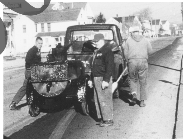
Village highway department crew at work on Carmen Street.
