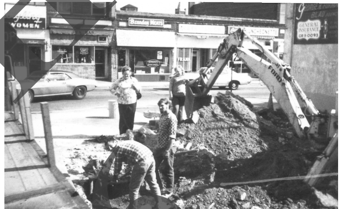
Highway department crew installing pumping station on Lake Street near Ocean Avenue. This section on North Ocean Avenue always had been prone to severe flooding.
