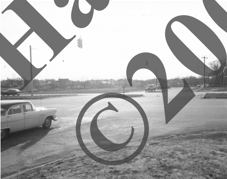
The intersection of Sunrise Highway and North Ocean Avenue in the 1950’s. The four lane Sunrise Highway had only grade crossings controlled by traffic lights in these years. With increased traffic the accident rates rose, and improvements were urgently needed.
