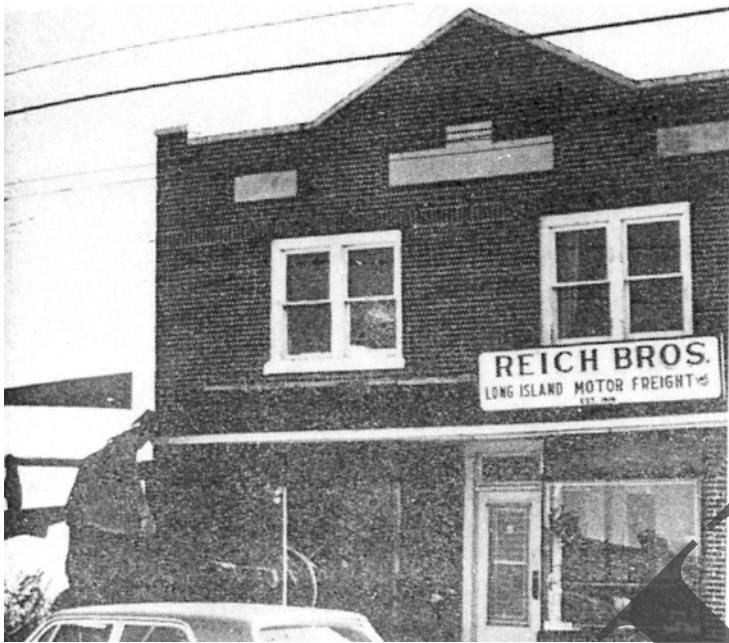
The Reich Brothers Trucking Company office building on the south side of East Main Street, between Evergreen and Grove Avenue, was built in 1928 and demolished in 1981, when the property was sold.
